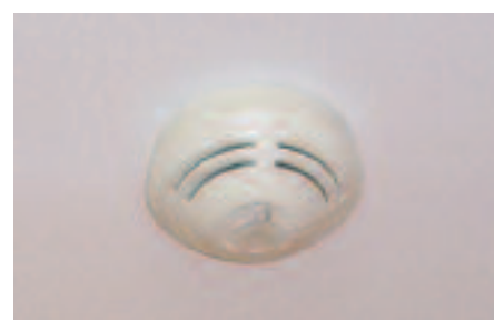
... as well as the IQ8Quad fire detectors.
